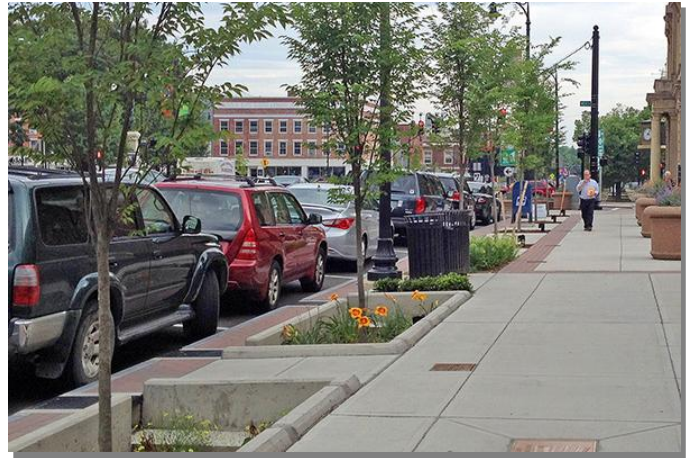
North Street, Pittsfield, MA. Bioretention Planters receive stormwater from the street and sidewalk. Photo courtesy of Vanasse Hagen Brustlin, Inc.
